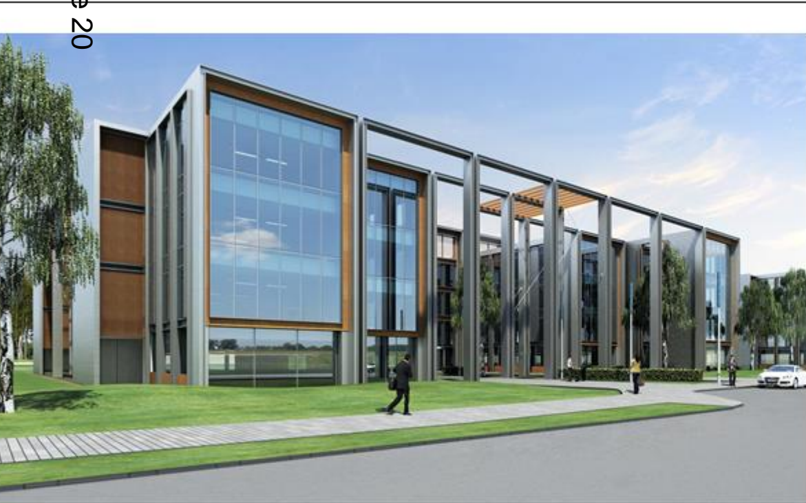
CGI 03 - Frontage to Pinehurst Road
